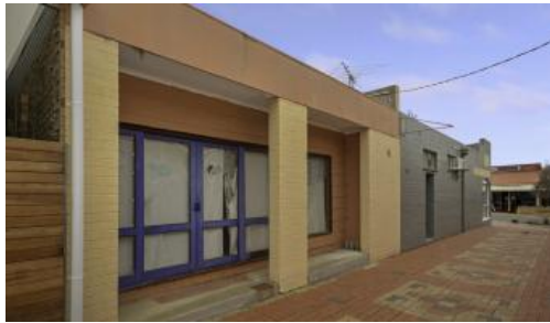
139 Main Street, Stawell
